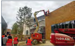
Construction du Shopping Promenade® de Claye-Souilly
