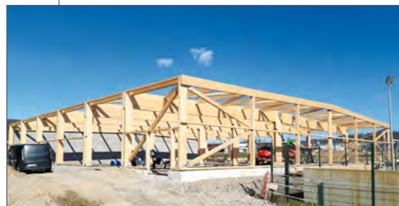
Green 7 (Salaise-sur-Sanne) is equipping its Basic Fit and Tool Station buildings with a superb 50-tonne wooden framework and 60-tonne wooden walls and cladding (pine and larch) from the French timber industry.
