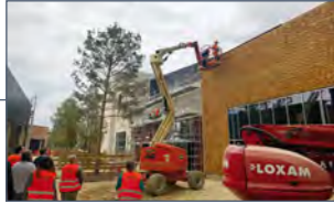
Construction of the Shopping Promenade® in Claye-Souilly
