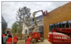
Construction of the Shopping Promenade® in Claye-Souilly
